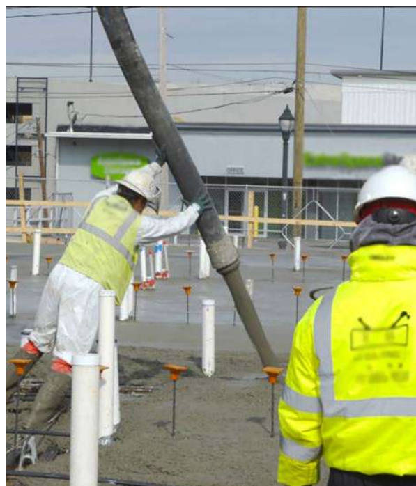
Carbon Dioxide Utilization. Captured CO 2 utilization in concrete (photo by Sustainable Energy Solutions).
