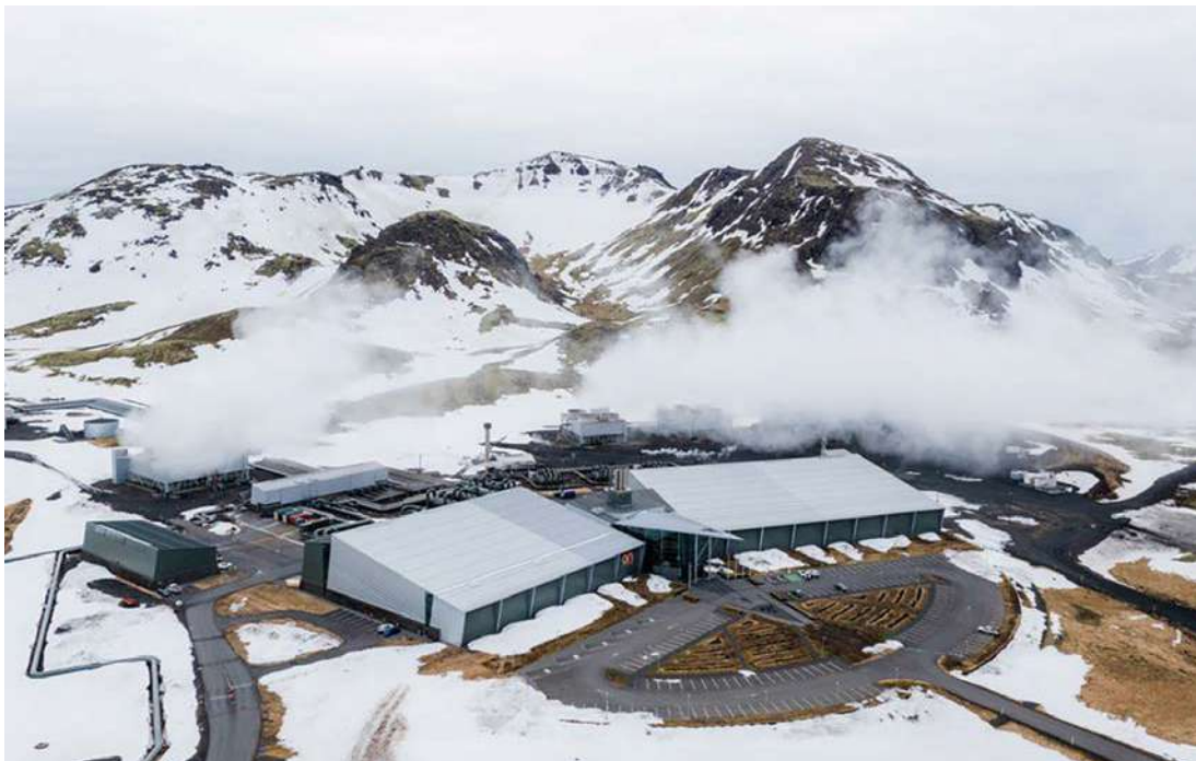
Carbfix flagship project. Carbon dioxide capture and mineral storage at the Hellisheidi Geothermal power plant in Iceland (photo by Carbfix).
